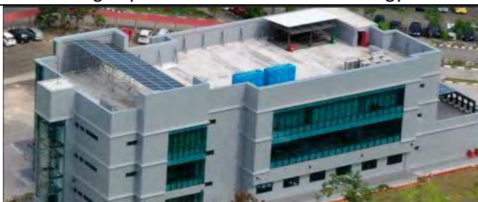
Example of Green Building Implementation – Renewable Energy
