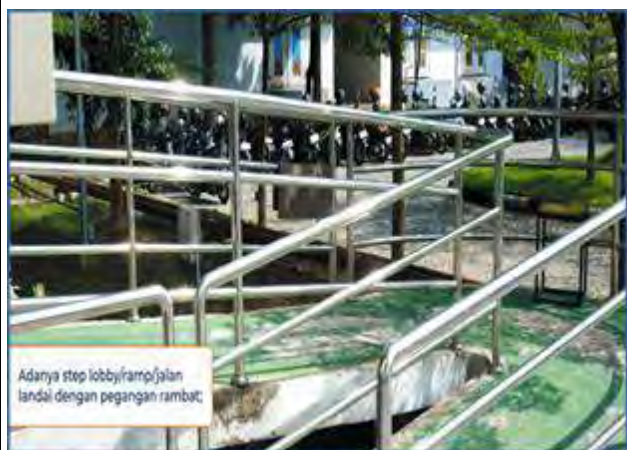
5. Accessible ramp with handrails
