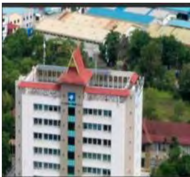
1. Renewable energy Main Building
