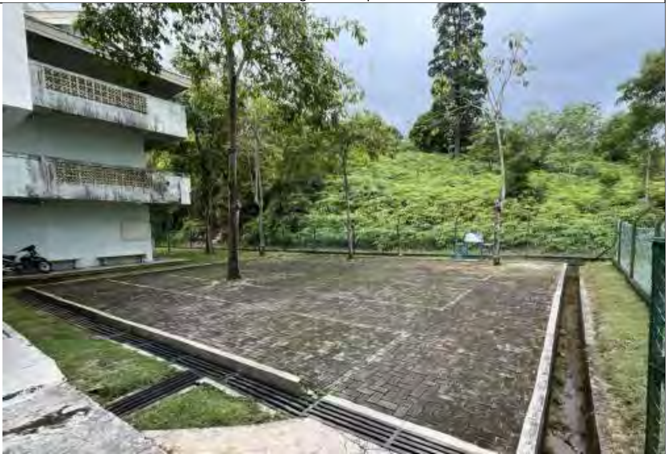
Parking Area Campus 2
