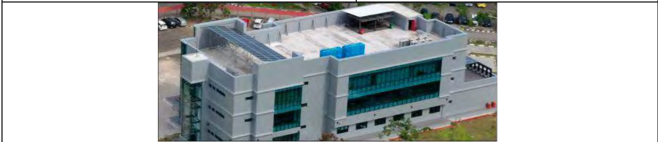
Example of Energy Efficient Appliances Usage: Solar absorption Air Conditioning system (Politeknik Negeri Batam, Batam)
