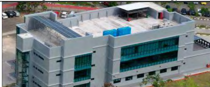
Example of Green Building Implementation – Renewable Energy
